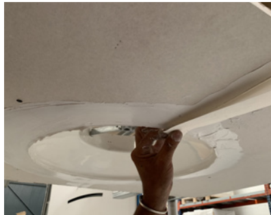
With application of "anti-cracking bandage".
