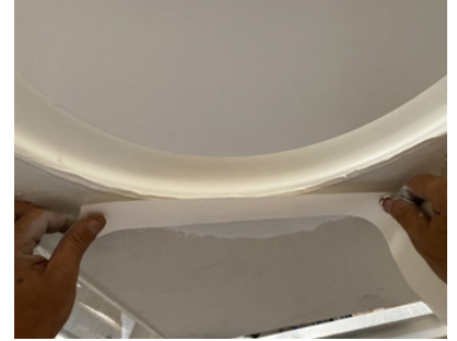
With application of "anti-cracking bandage".
