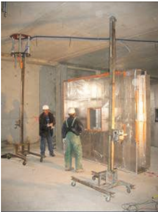
1 - Place the panel in its position
