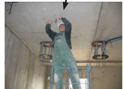
2. Place the anchor plug
