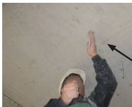
3. Insert the rod in the block
