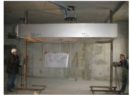
3 - Raise the panel simultaneously to its position, making sure that the rods are properly inserted into the anchorage points
