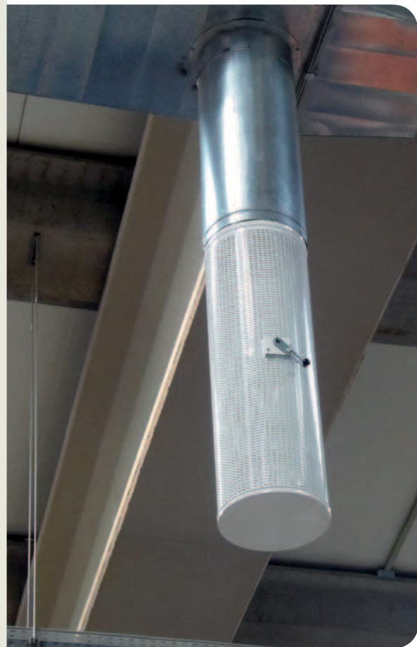
S90-GV, nave industrial
