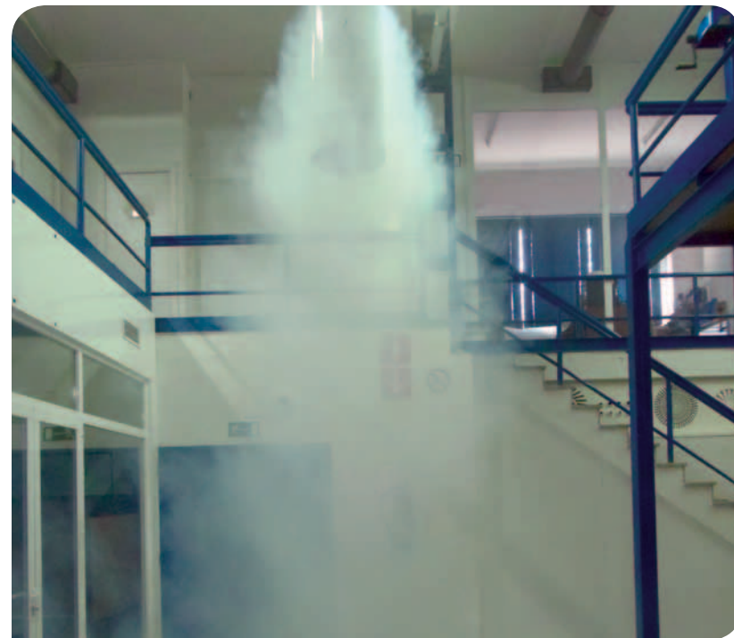
S90-GV, nave industrial
